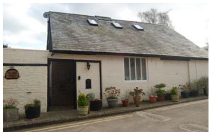
Photo 98: The Old Forge, Pit Lane
