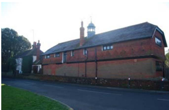
Photo 121: Littlemead and Paddock Cottage, formerly part of Grange Farm, turn their backs on the road.
