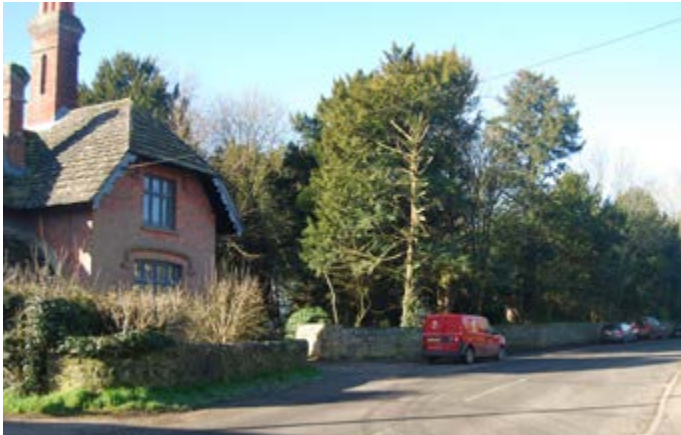
Photo 126: The stone and flint wall with overhanging trees along the frontage to Pakyns Manor
