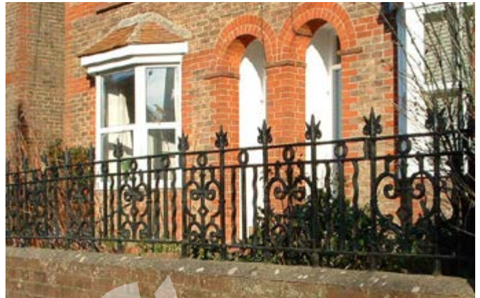
Photo 115: Decorative iron railings topping boundary walls to the north of the Area
