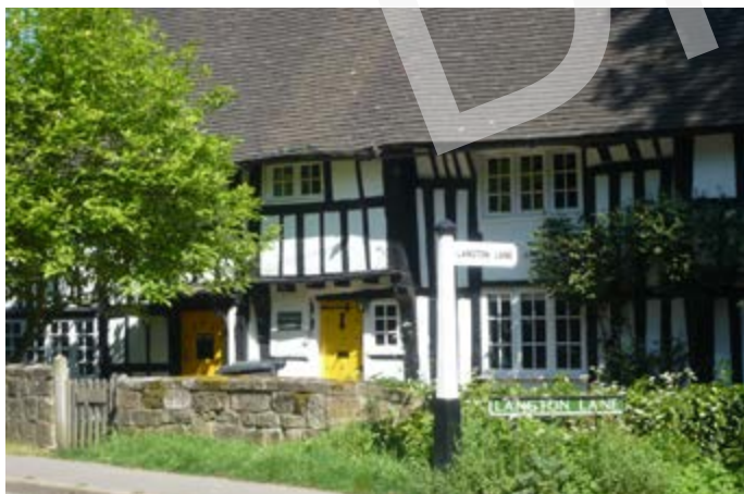
Photo 7: Tott Farmhouse, Tott Lane- a 16th century three storey timber framed house, refronted with stucco and tile hung.
