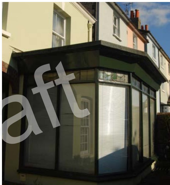
Photo 40: The shopfront at 17 High Street
