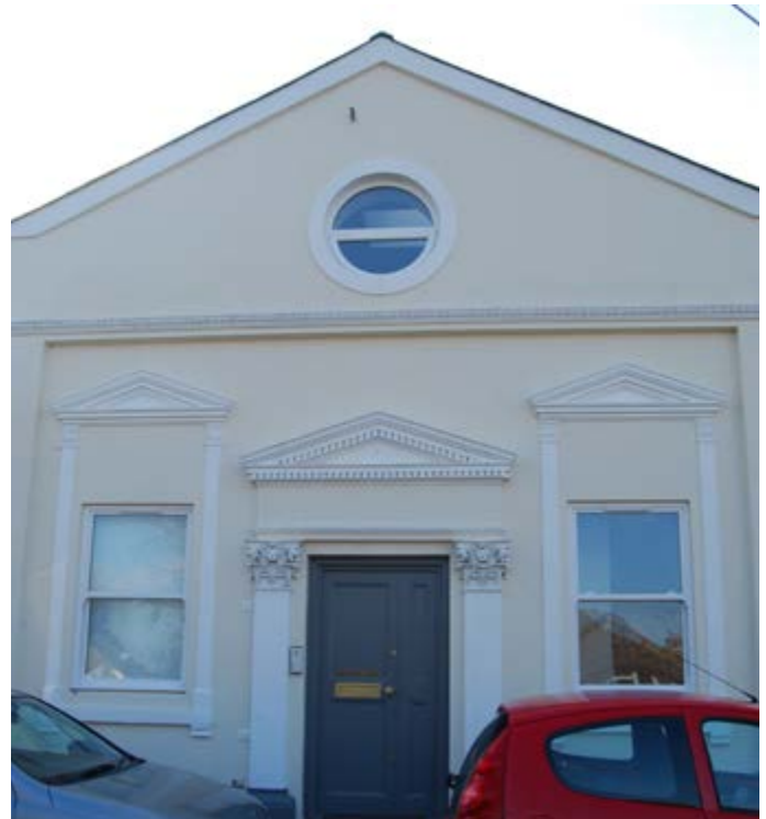
Photo: 11 The former Methodist Chapel on Manor Road
